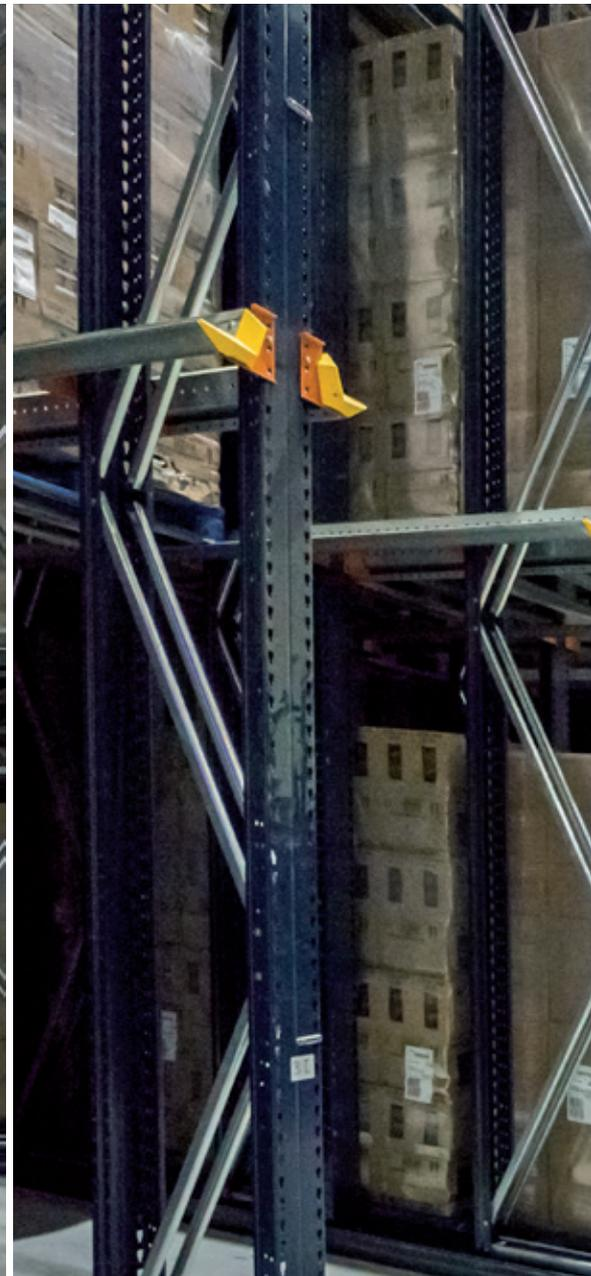
simplifying pallet truck manoeuvres and preventing blows against the rack structure.
