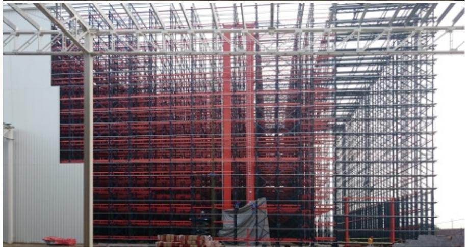
Tubes in the fire safety system are installed and fixed to the racking, thus shielded from occasional impacts and enabled to spray pallets properly in case a fire breaks out
