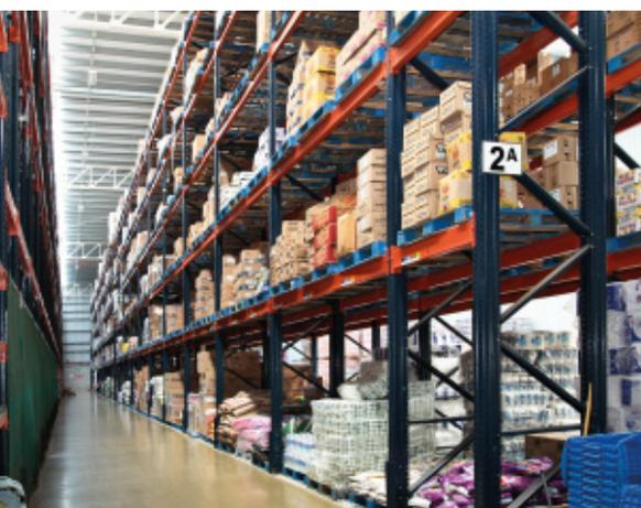
The picking towers can store 1,908 pallets all together in the live racking, 2,840 pallets in the push-back ones and 40,700 cardboard boxes
