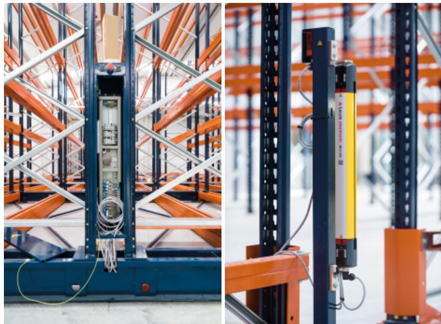
The Movirack units incorporate safety devices, such as external and internal barriers with photocells, which stop all activity when operators work inside the aisle
