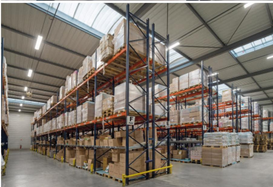
Pet food master Royal Canin owns and operates a warehouse comprising the pallet rack storing system by Mecalux. Some lower storage shelves of the racks have live channels set up in them for smooth picking of smaller sized products. So, the installation has a full consolidation area, enabled with conveyor units.
