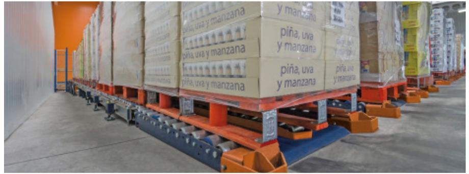
The facility was set up to handle and store medium sized pallets since the percentage, compared to euro-pallets, is higher
