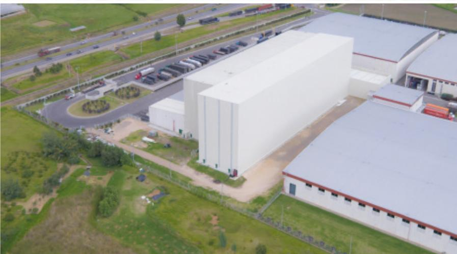
Grupo Familia, a company specialising in personal care and hygiene products, has a 35 m high automated clad-rack warehouse capable of handling around 17,000 pallets. In the supply of the warehouse, located in the Colombian municipality of Cajicá, Mecalux has also included the Easy WMS warehouse management system and the Galileo control programme, which are tasked with monitoring and executing the movements related to the logistics process.
